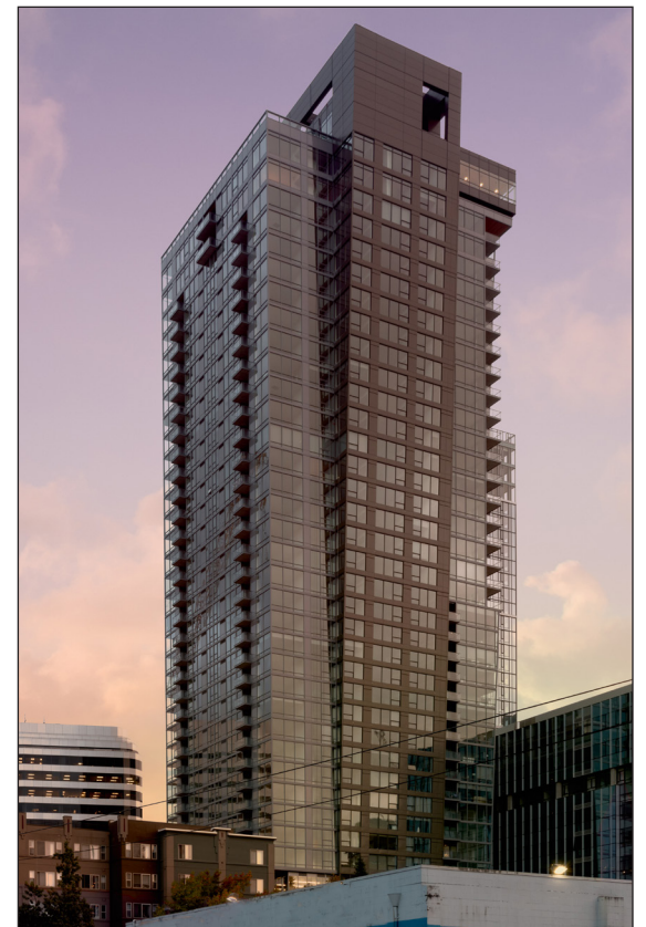
Three sides of the tower taper outward as the building rises. The floor plate on level 39 is 50 percent larger than the floor plate on level eight.
